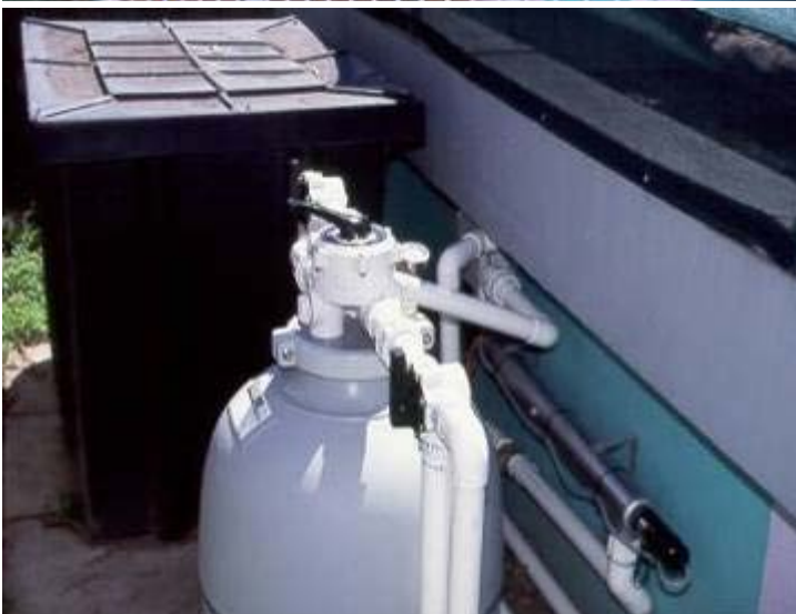
Three types of filtration- Mechanical (Grey pond filter), Biological (black tub with dense matting) and UV Clarification/Sterilisation (Stainless steel tube)
